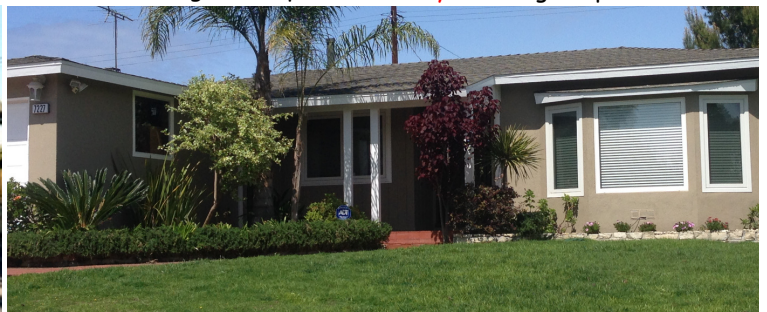
April/May: New roof and paint job for our Los Angeles house
